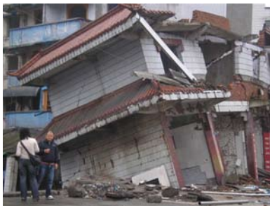
Quake damage in Hanwang in China's Sichuan Province.
